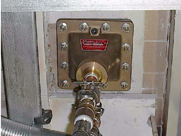
OXY-THERM® LE mounted on a glass furnace
